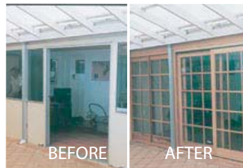
Stegbar Installation Service
